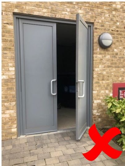
Fig 5 Double doors do not stay open and swing shut fast, hindering collections
