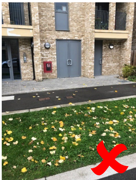
Fig 10 Swales mean there is no smooth access from bin store & bins have to be dragged across grass
