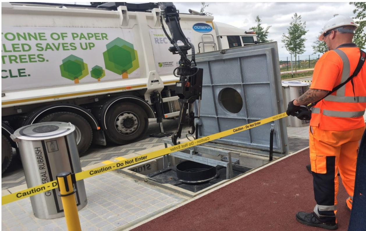
Fig 19 Underground bins hook-lift system in the ground
