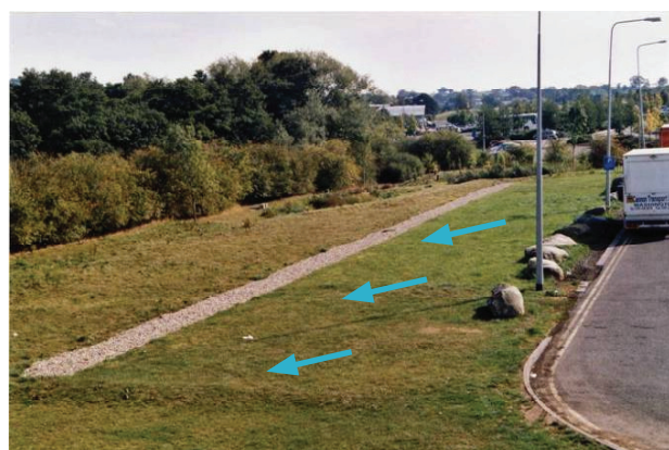
Filter strip leading to a filter drain. The filter strip removes silt and reduces the maintenance required for the filter drain, Hopwood services, M42
